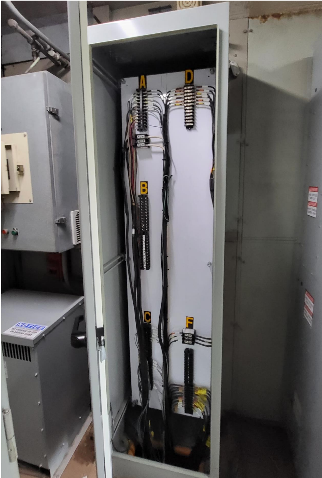
CT4 indoor junction box (opened) after installation
